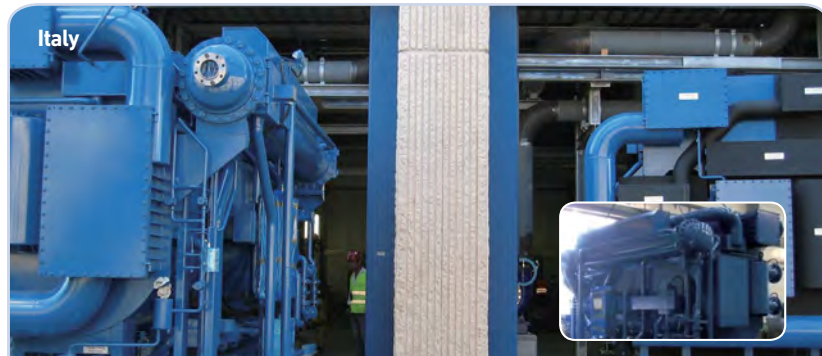
3SUN Group Co-generation Plant in Catania SW & 2AB 2,388 usRT(8,396kW)
