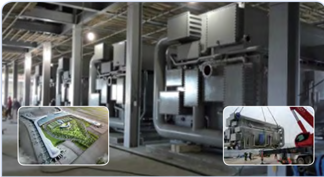
Incheon Interational Airport 2AB 8 sets 8,000usRT(28,128kW)
