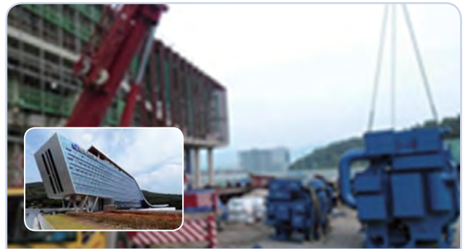
Korea Gas Corporation Daegu Office 2AB 1,300usRT(4,571kW)
