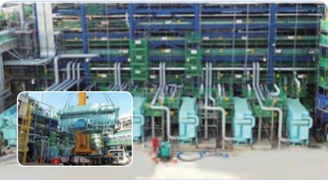
Samsung Total SW & HWAR-L 9,787usRT(34,411kW)
