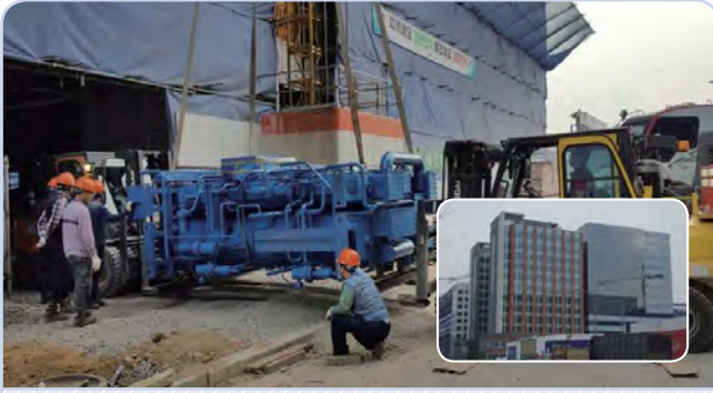
Hwaeom Building Munjeong-dong 2AB 270usRT(949kW)
